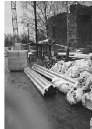
Figure 3.21 Air ducts at a construction site (left) can cause considerable air pollution indoors after installation, caused by accumulated dust/debris; capping the ducts (right) is a good solution
