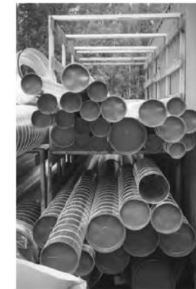
Figure 3.21 Air ducts at a construction site (left) can cause considerable air pollution indoors after installation, caused by accumulated dust/debris; capping the ducts (right) is a good solution
